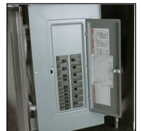
Breaker panels are factory wired and tested
