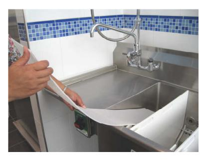
Begin bending the flow guide to the shape of the front rib set, and allow the notches of the flow guide to engage the hooks of the rear rib set.
