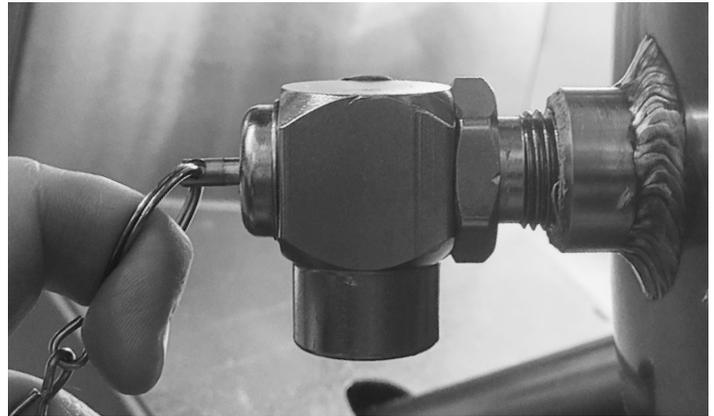
Test the operation of the safety valve on a regular basis.
