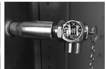
The open end of the pressure relief valve must face downward.
