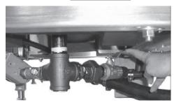
The manual drain valve is located under the boiler. Whenever the boiler is turned off and allowed to cool to about 130°F, it drains automatically. This should be done every day to minimize scale buildup inside the boiler.
