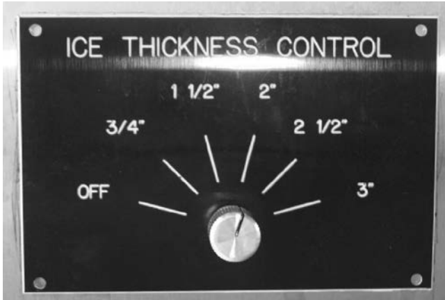
Ice Water Thickness Control Panel
