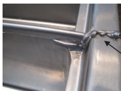
APPLY THE GREY-COLORED NSF APPROVED SEALANT TO ALL THE SINK JOINTS AND WIPE THE EXCESS AWAY LEAVING A SMOOTH SANITARY JOINT.
